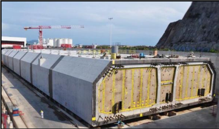
IMMERSED TUBE TUNNEL UNDER CONSTRUCTION
