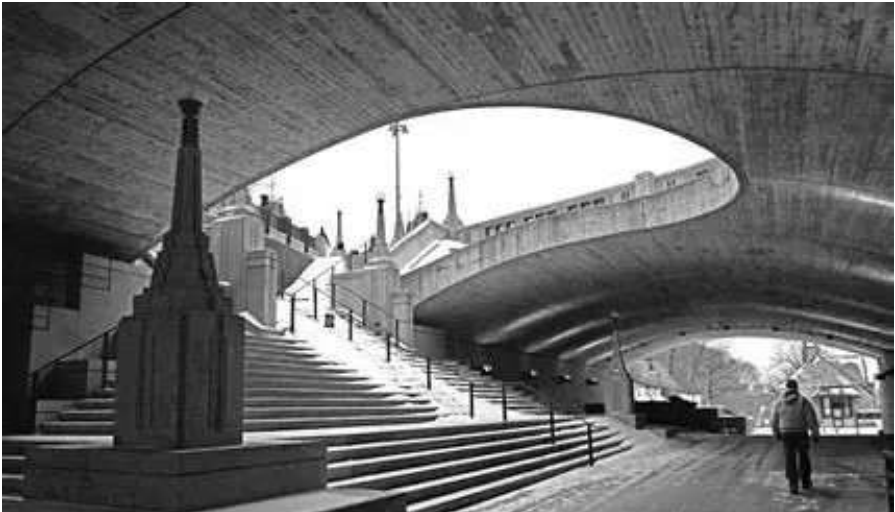
A pedestrian environment open to daylight with a flowing form is a creative and unique space. Open lines of sight enhance security. This is a pedestrian setting from Ottawa.
